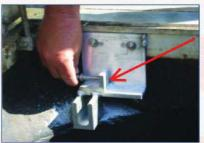
Install (2) 3/8" x 1  $^{1}$ /2" pivot bolts from the outside to inside of both pivot clevises until the end of the bolt is flush with the inside of each clevis. (Do not install the bolts past the inside edge of the clevis). The Retro-Grate<sup>TM</sup> will be positioned between the two pivot clevises and clearance for the grating structure must be maintained.
