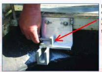
Install (2) 3/8" x 1 1/2" pivot bolts from the outside to inside of both pivot clevises until the end of the bolt is flush with the inside of each clevis. (Do not install the bolts past the inside edge of the clevis). The Retro-Grate™ will be positioned between the two pivot clevises and clearance for the grating structure must be maintained.
